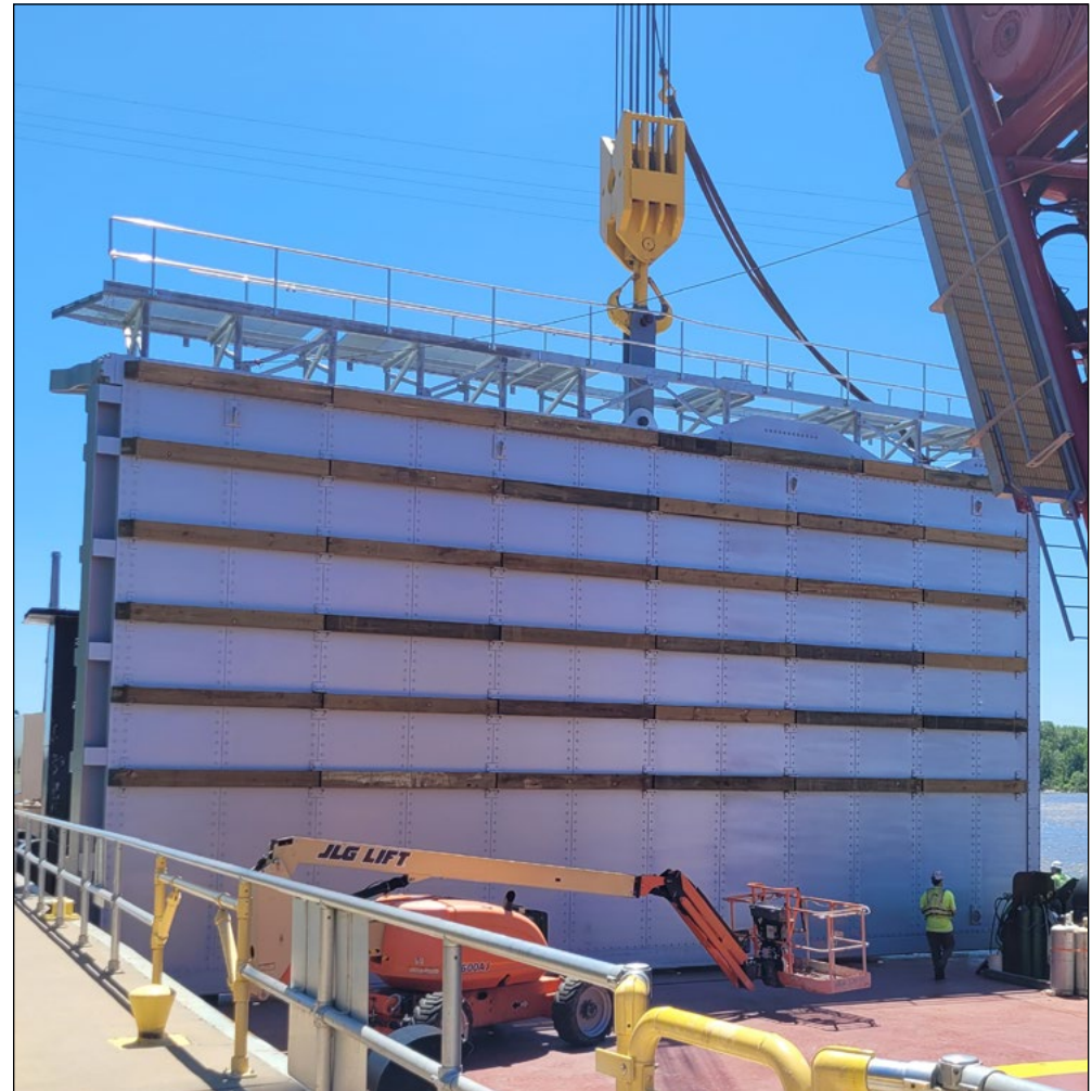
Maintenance and repair crews from the St. Paul and Rock Island Districts install a new 121-ton miter gate at Lock and Dam 8 near Genoa, Wisconsin, June 16. USACE St. Paul District photo by Melanie Peterson
